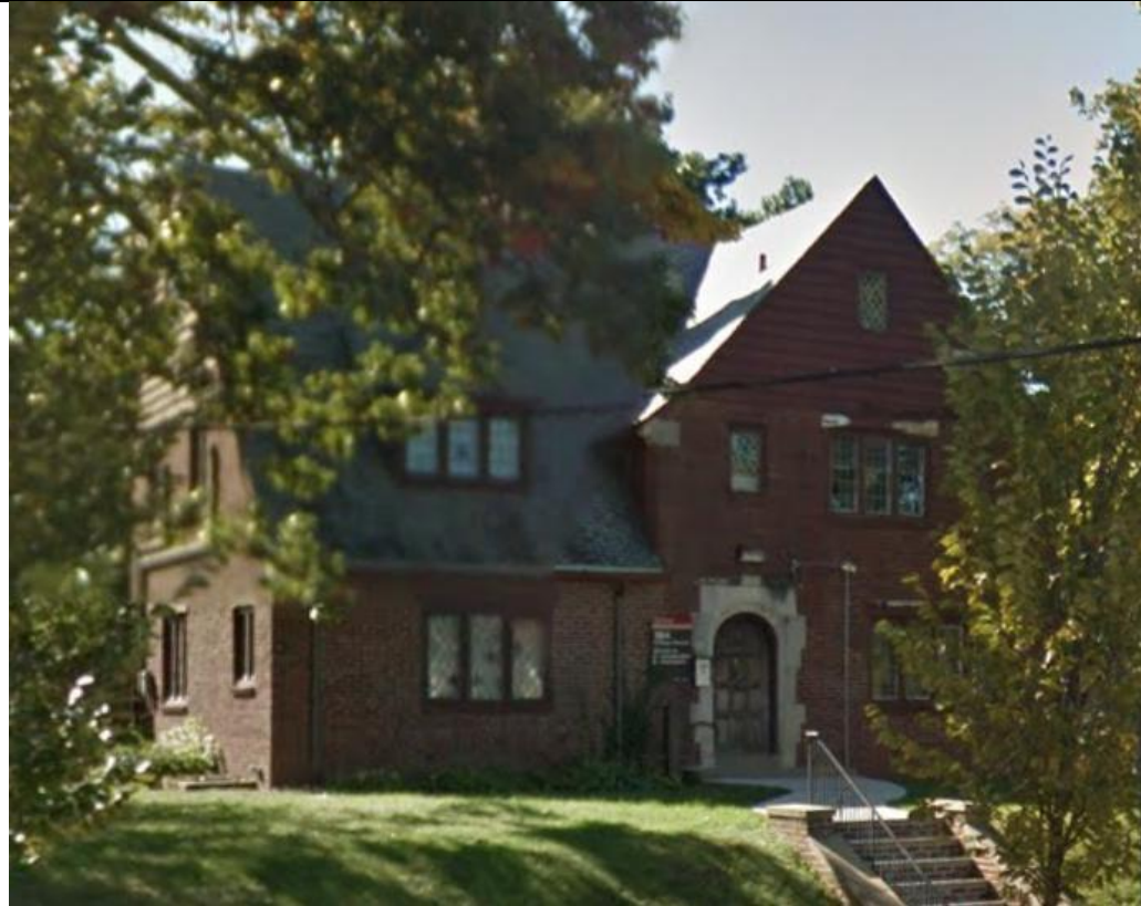
Huntington House, another former private home that has been converted to a building with a meeting room, doctoral student lounge, and faculty offices, was acquired by the school in the early 2000s.
